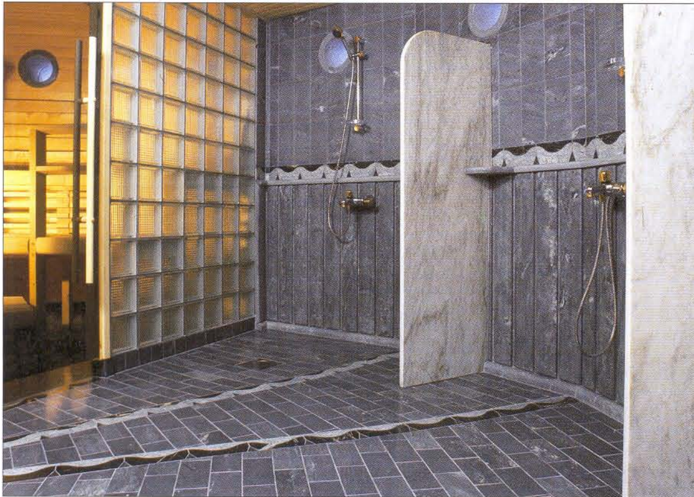
Floor and walls, Kianta Blue. Abrasive water jet border strips, Kianta Black and Tulikivi Classic. Shower walls, marble.
